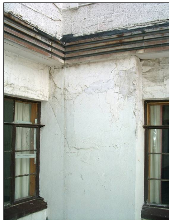
Cracks in stucco should be repaired to avoid moisture entering and enlarging them.
