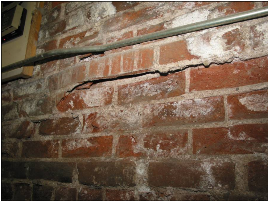
Efflorescence, a white chalky surface residue, indicates the presence of moisture and can cause significant deterioration of masonry.
