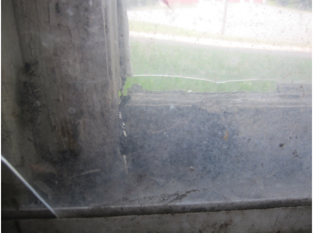
Figure 6. Window at northeast corner of basement. Not only is the pane broken, but there is separation of the stile and rail, and rot.
