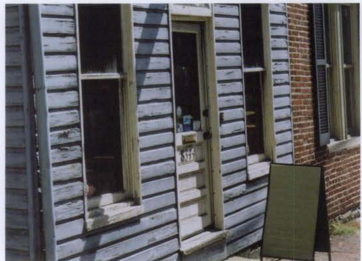
Figure 8. The paint on the siding of this south-facing wall needs to be scraped, sanded, primed and repainted. Postponing such work will lead to further paint failure, require greater preparatory costs, and could even result in the need to replace some siding. Photo: Charles Fisher.
