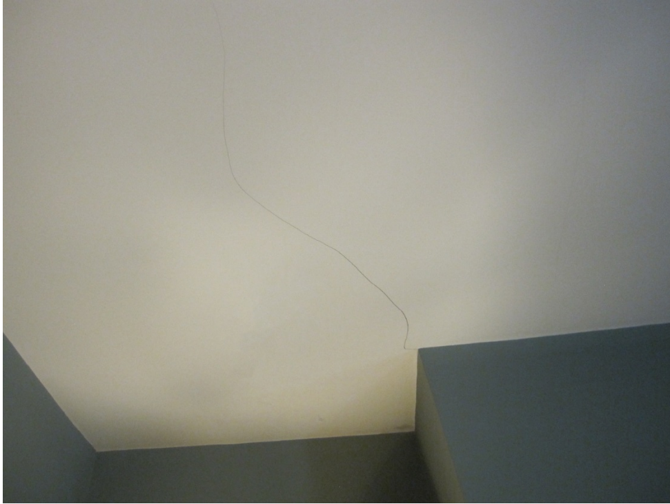
Figure 12. Ceiling Crack in northeast room. There is no associated water damage.
