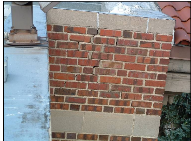
Masonry parapet walls are prone to moisture damage, such as deteriorated mortar joints, and should be examined regularly.
