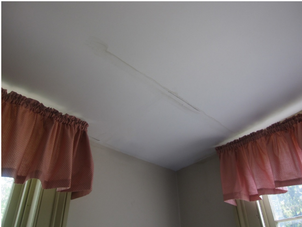
Figure 13. Ceiling Crack in southeast room. This crack has associated water damage as indicated by the staining.
