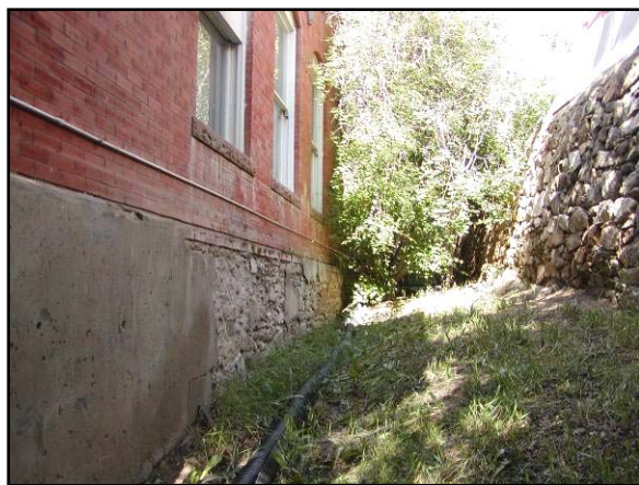
Ground that slopes towards the building foundation will bring unwanted moisture and should be addressed.
